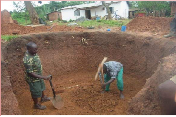
An image showing the excavation work after lay out
