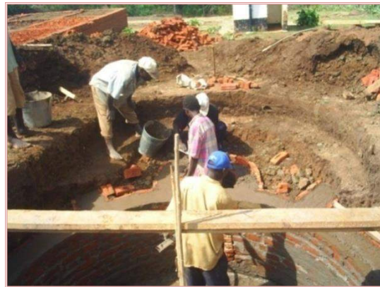
Right: Digester walls being built.
