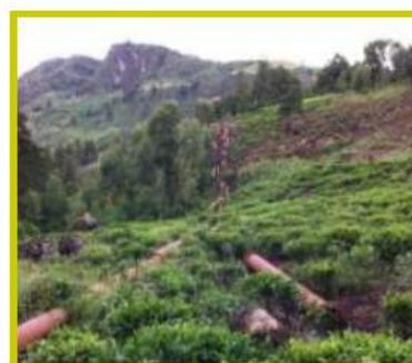
Pipes waiting to connect powerhouse to canal
