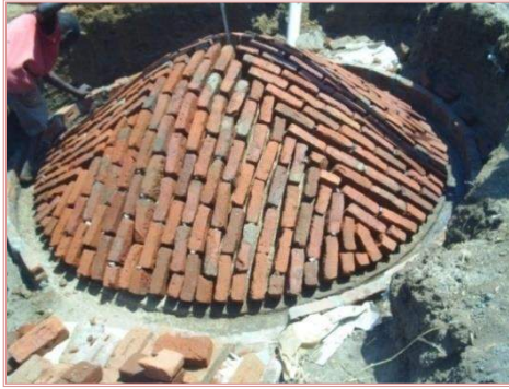
Fixed dome being constructed
