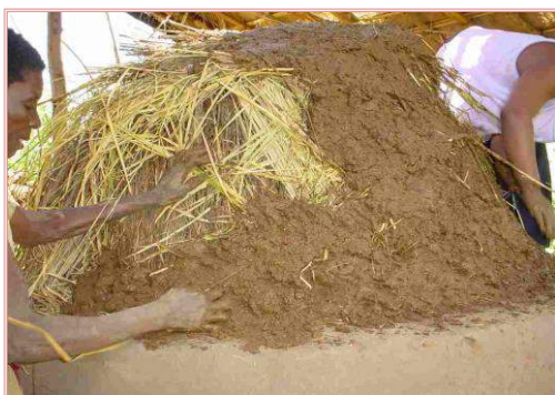
Smear with soil to cover grass
