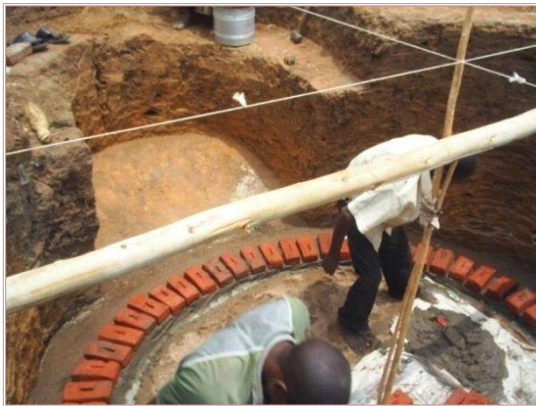
Left: Biogas digester foundation being built.
